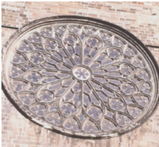
Fig. 3a. View of the rose window in the main façade of the church of Santa María del Pi in the Cita Vella of Barcelona. The construction and symmetry is very similar to the one found in the upper rose window at the main entrance to Reims Cathedral in France. From the central 6-fold repeat the number of ‘rays’ doubles (left-right) as it expands out to 12 ‘petals’ and contains 24 curved triangles on the outmost edge. Ignoring the innermost hexagon, the rose has symmetry C_{12v} (12 mm). Image from the author’s personal collection.
